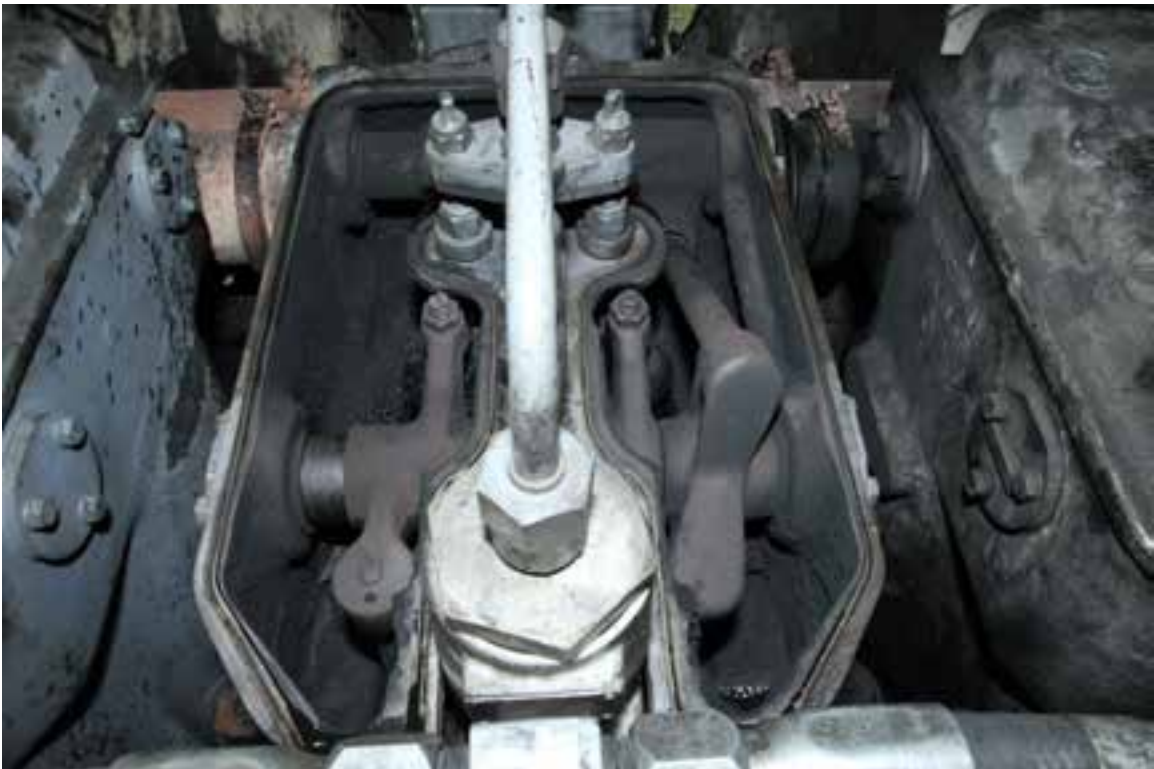
Figure 4: Power assembly R5 showing dry, coked valve train
