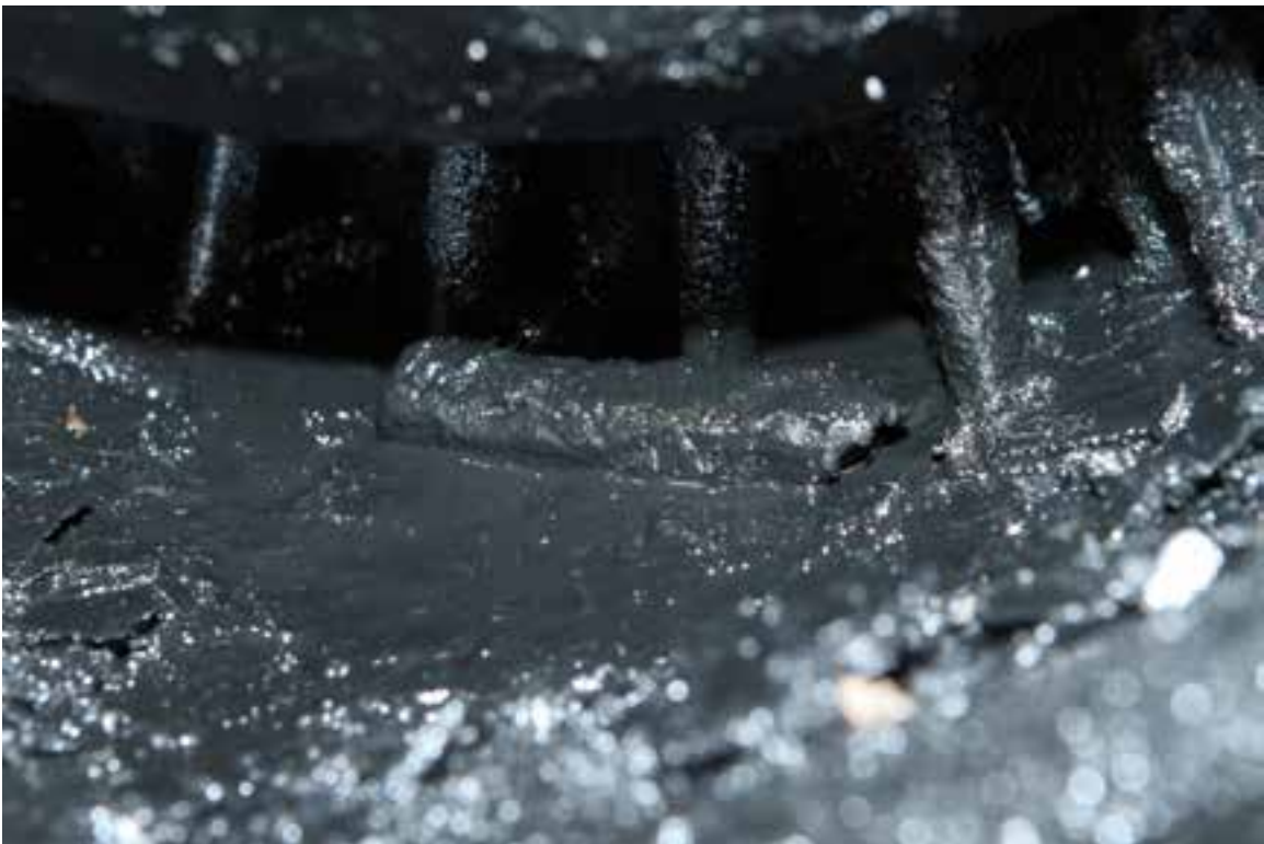
Figure 28: Portion of valve stem found just upstream of the turbine
