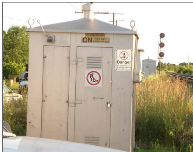
Photo 3. Signal bungalow with emergency signage
