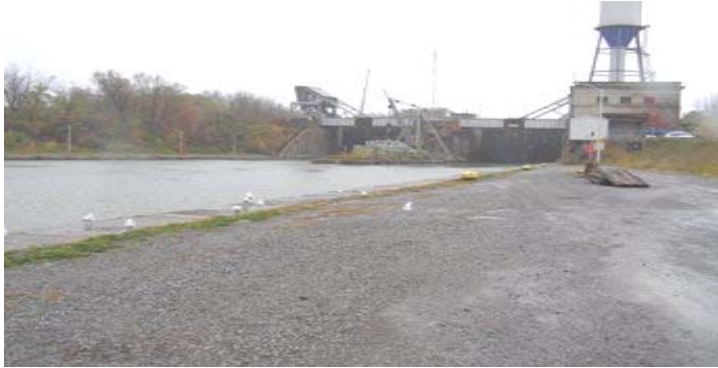
Photo 3. Lock 4, looking upbound (towards Lock 5)
