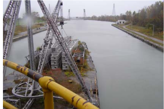
Photo 4. Bullnose, looking downbound towards Lock 3
