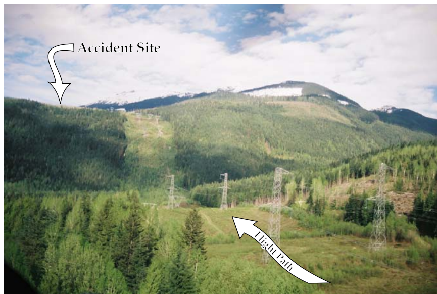
Figure 2. Powerlines leading to the accident site
